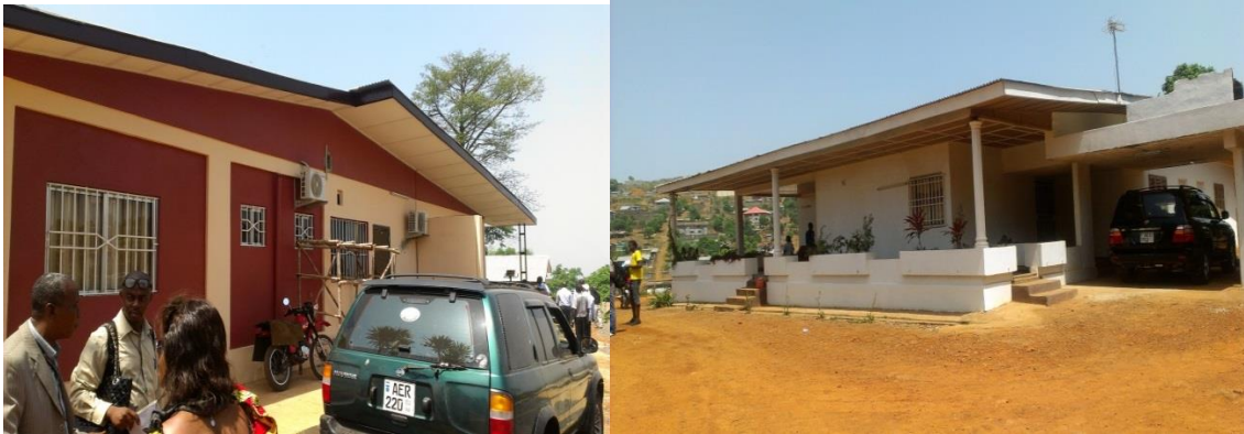
Figure 7. Refurbished villas by tenants
