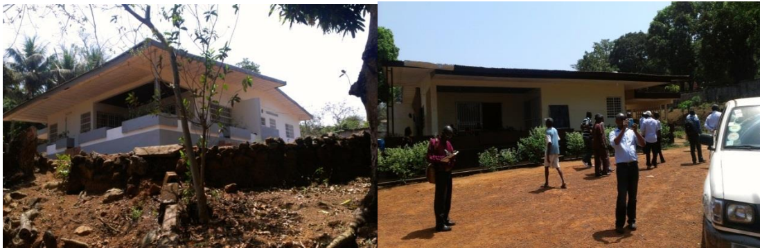
Figure 8. Refurbished villas by tenants
